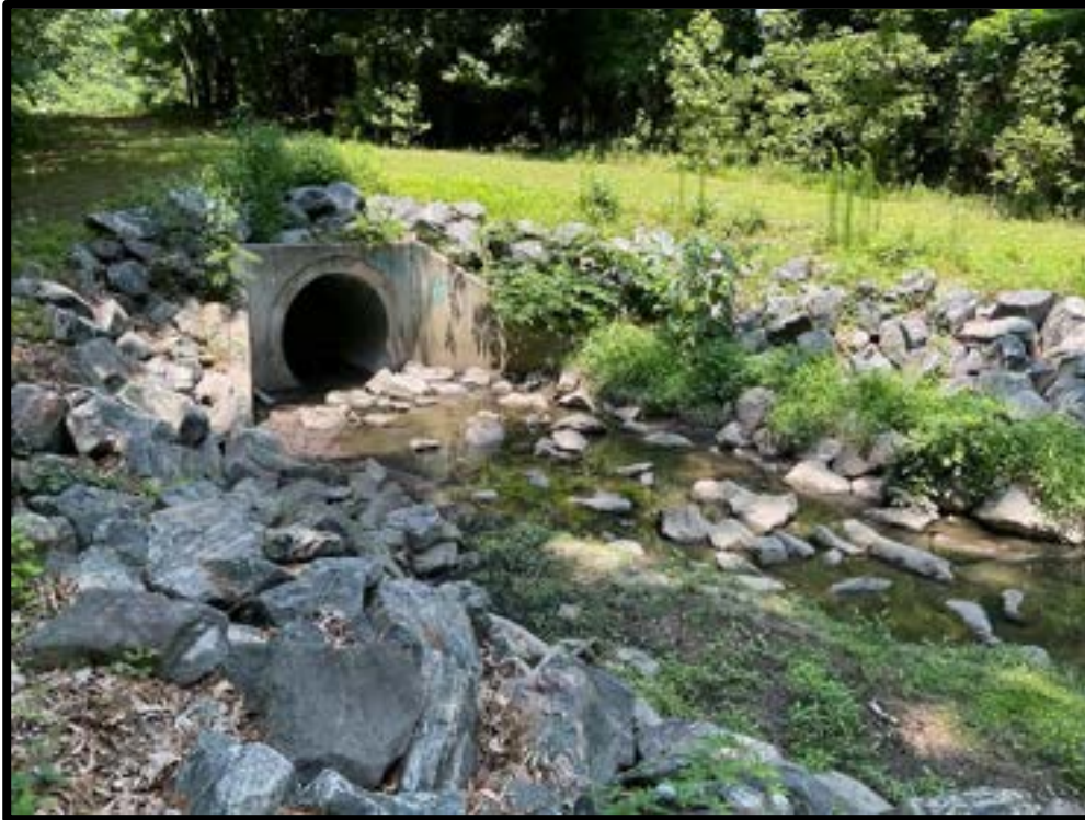
Photo #1: 72" Concrete Pipe
