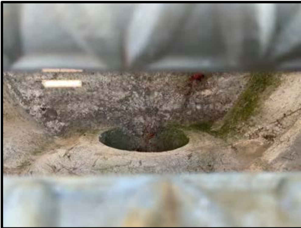
Photo #2: Some sedimentation present at upstream outfall pipe
