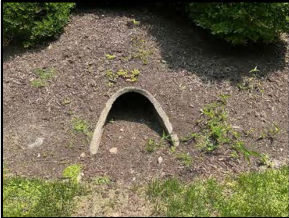
Photo #3: Sediment and vegetation accumulation present in southern inlet pipe and protection
