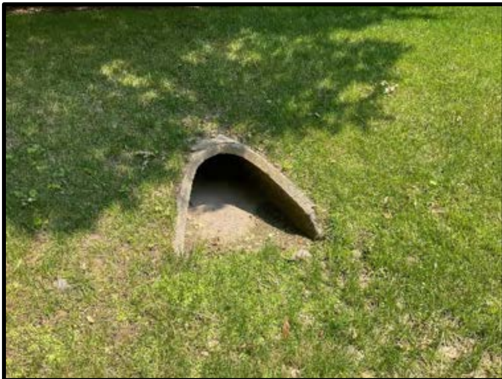
Photo #4: Sediment accumulation present in eastern inlet pipe
