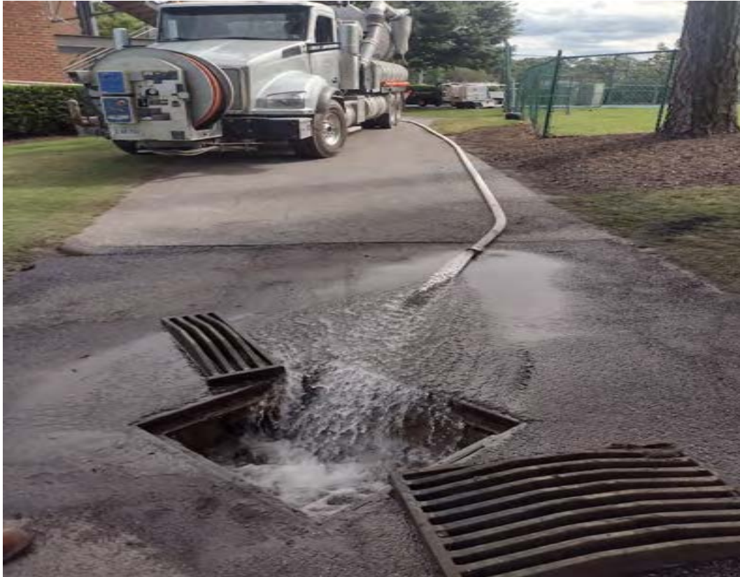
Vacuuming at Drain 3
