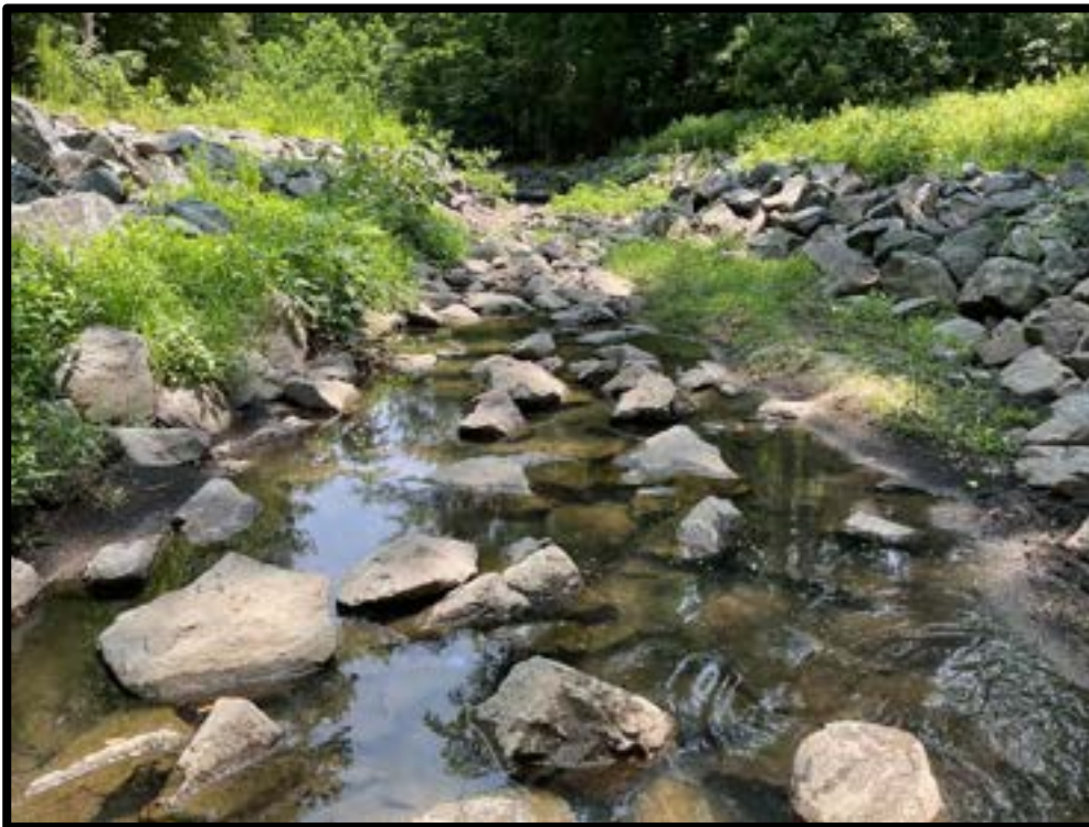
Photo #2: Outfall 3 receiving channel
