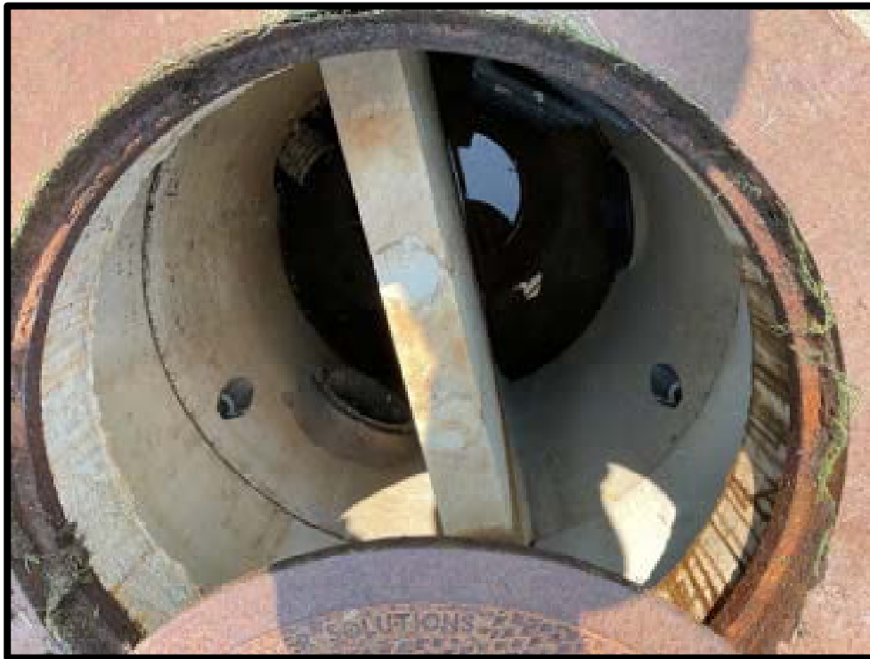
Photo #3: Southern structure appears to be in good condition
