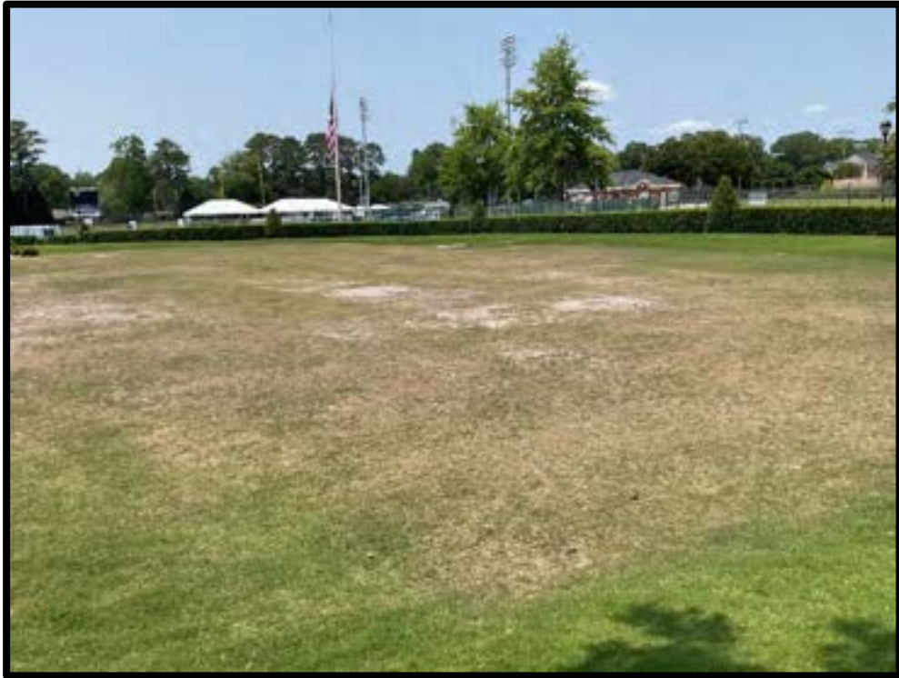
Photo #2: Bare areas present in bioretention
