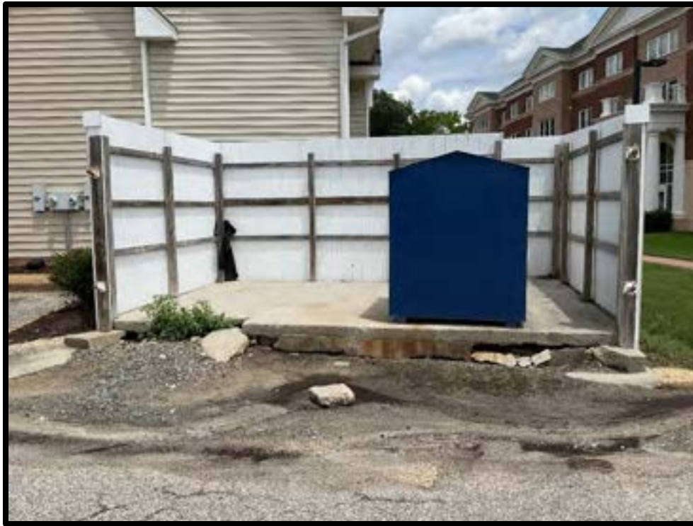
Photo #1: Significant road grit accumulation and concrete pad damage
