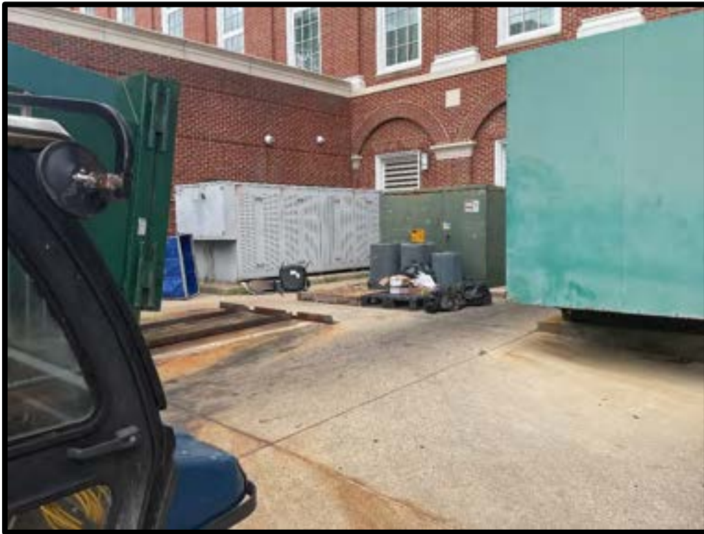
Photo #7: Container and materials storage
