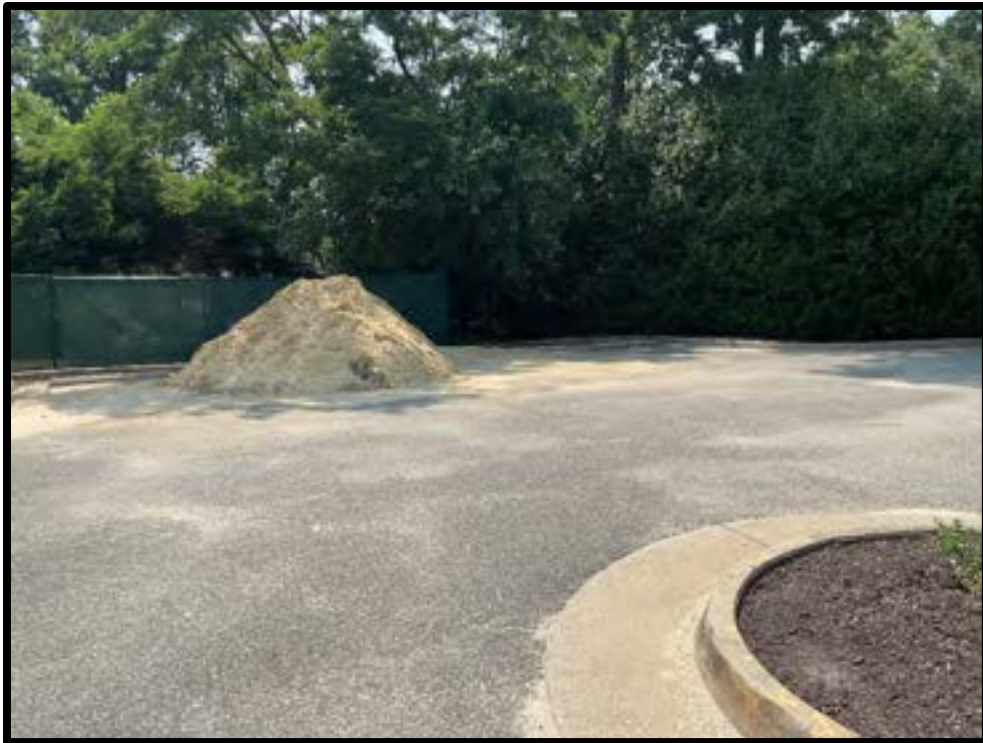
Photo #1: Uncovered stockpile
