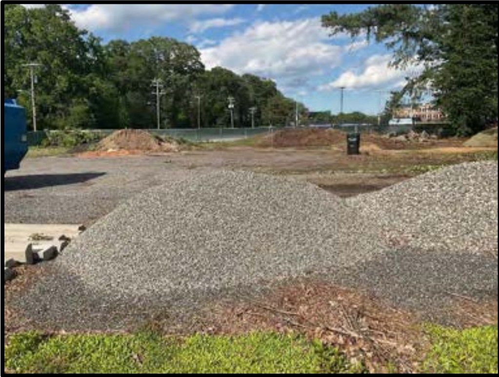
Photo #7: Uncovered stockpiles near receptacle area
