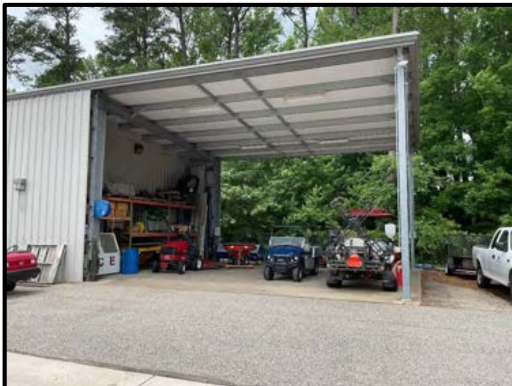
Photo #9: Covered equipment, materials, and storage area
