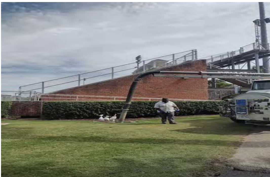
Vacuuming at Drain 3
