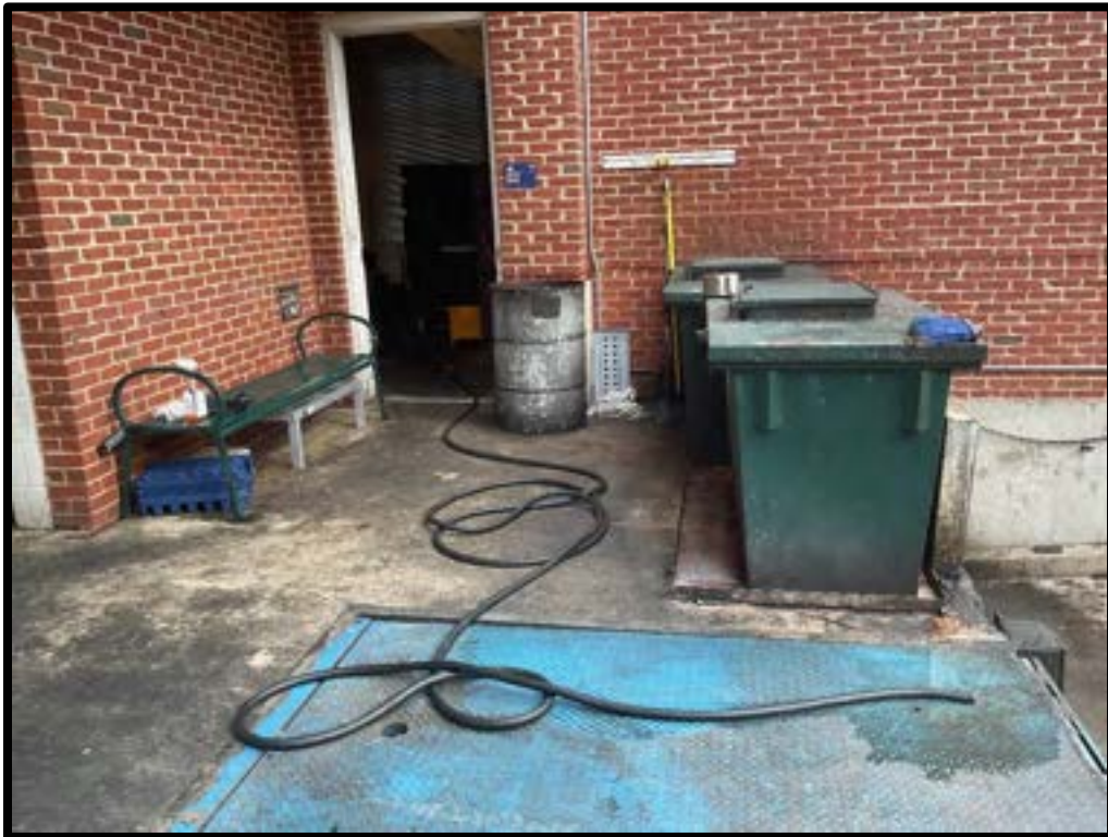
Photo #5: Hose discharging from inside building
