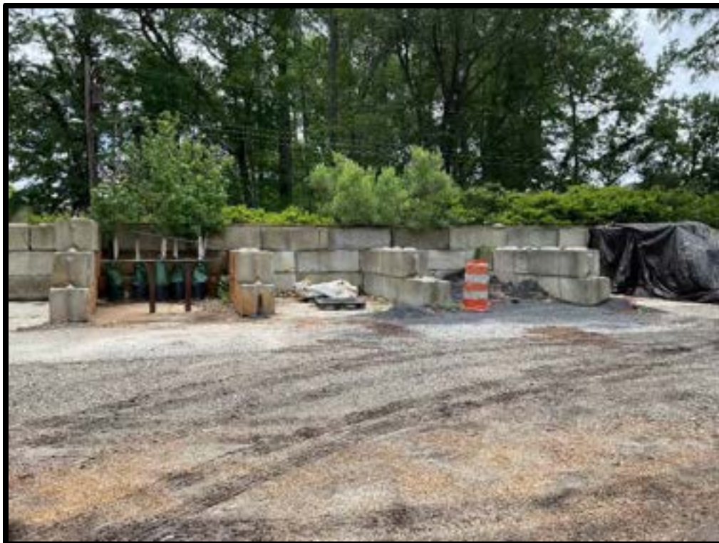
Photo #1: Partially covered and contained stockpiles
