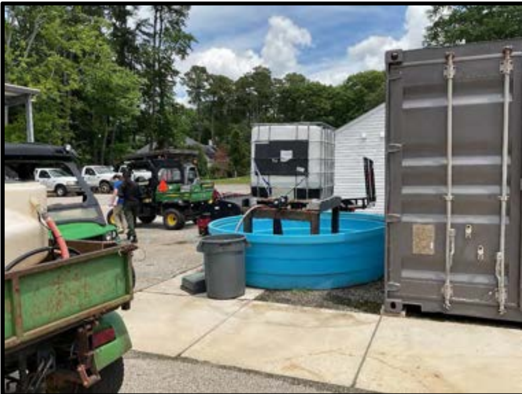
Photo #11: Elevated containers in secondary containment
