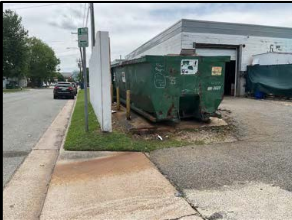
Photo #9: Rust stains and active discharge from dumpster
