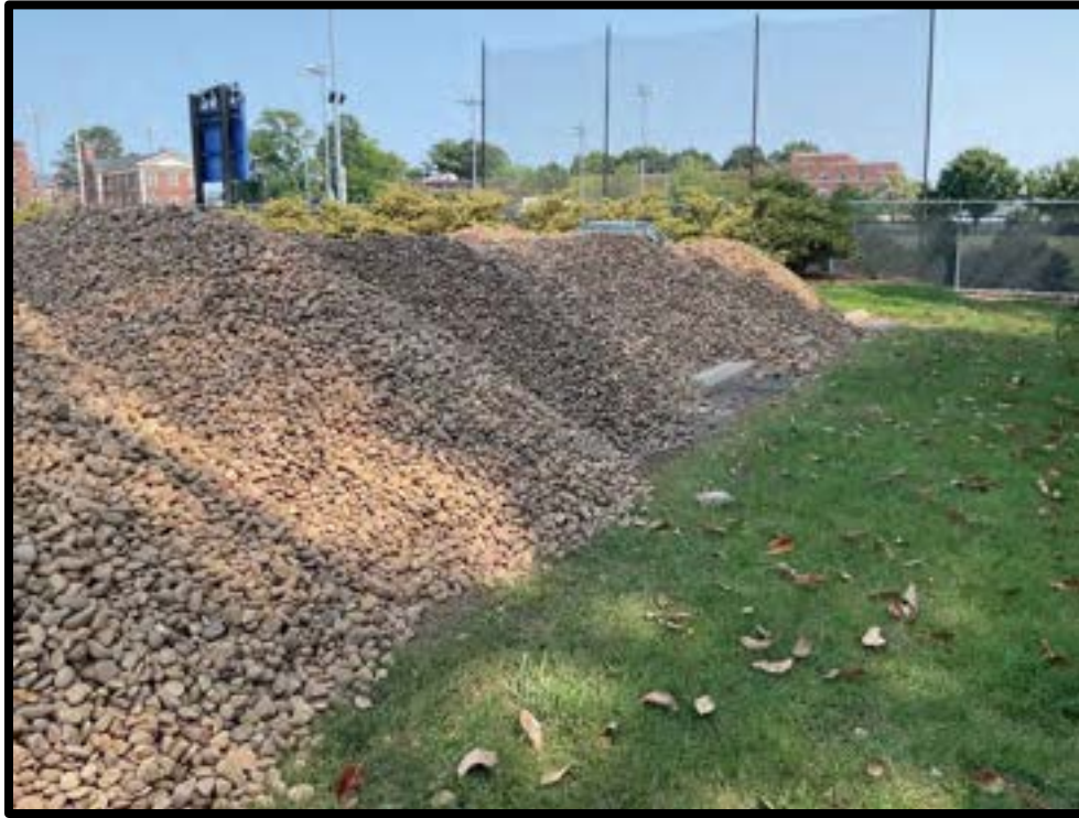
Photo #3: Back side of uncovered stockpiles
