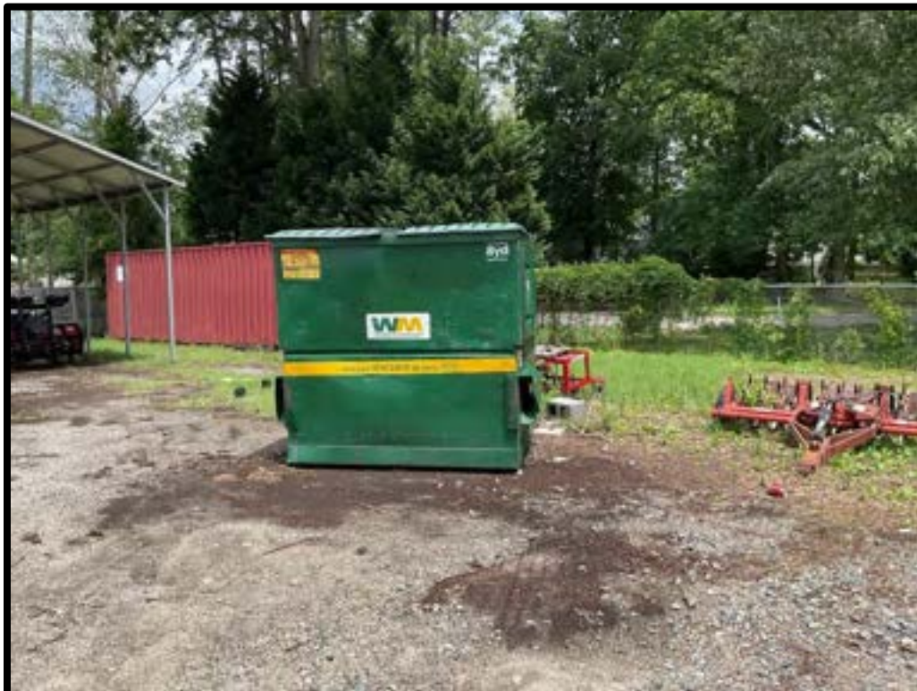
Photo #7: Covered dumpster with no secondary containment
