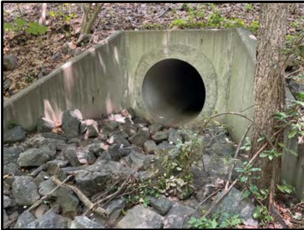
Photo #1: 48" Concrete Pipe
