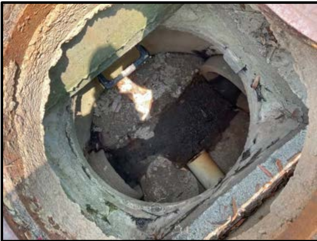
Photo #5: Some debris accumulation present in underdrain outlet pipe
