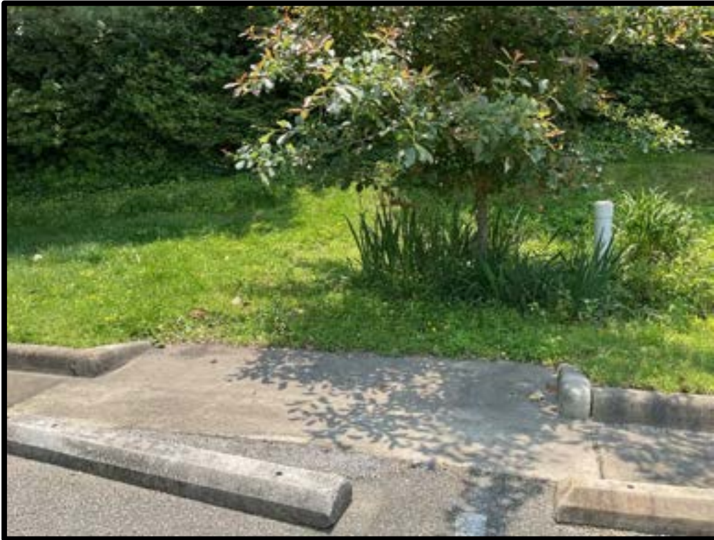
Photo #4: Northeast curb cut inlet appears to be in good condition
