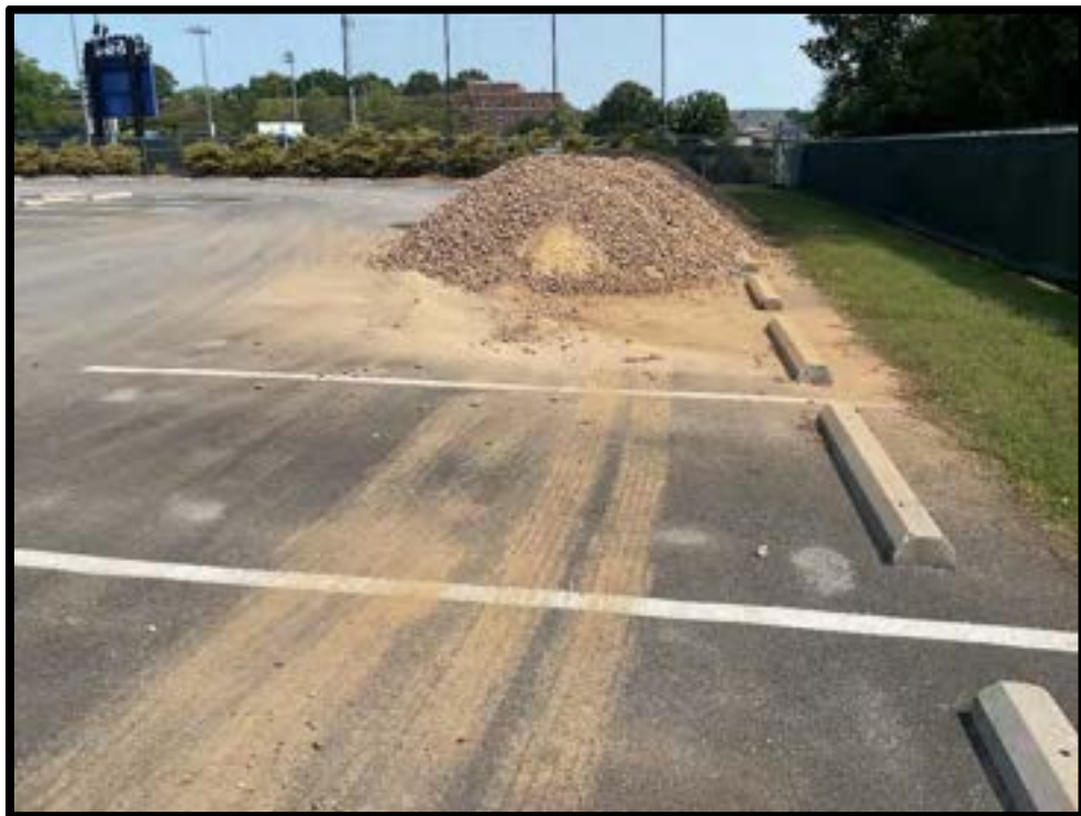
Photo #2: Sediment tracking onto parking lot from active baseball field operations
