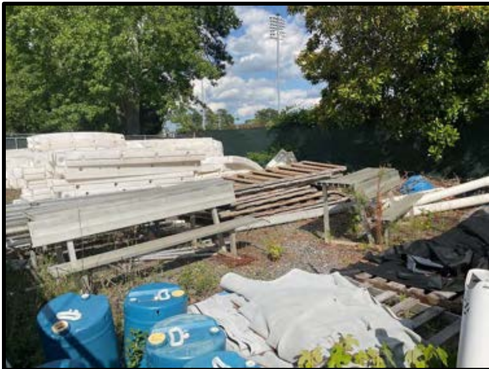
Photo #6: Uncovered materials storage area
