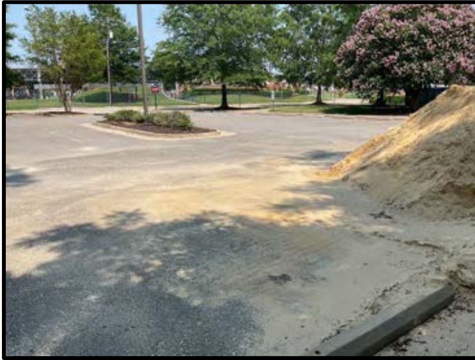
Photo #3: Sediment tracking onto parking lot from baseball field operations
