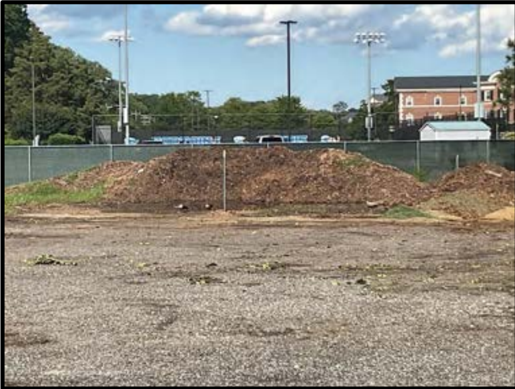
Photo #9: Ponding present near uncovered stockpiles
