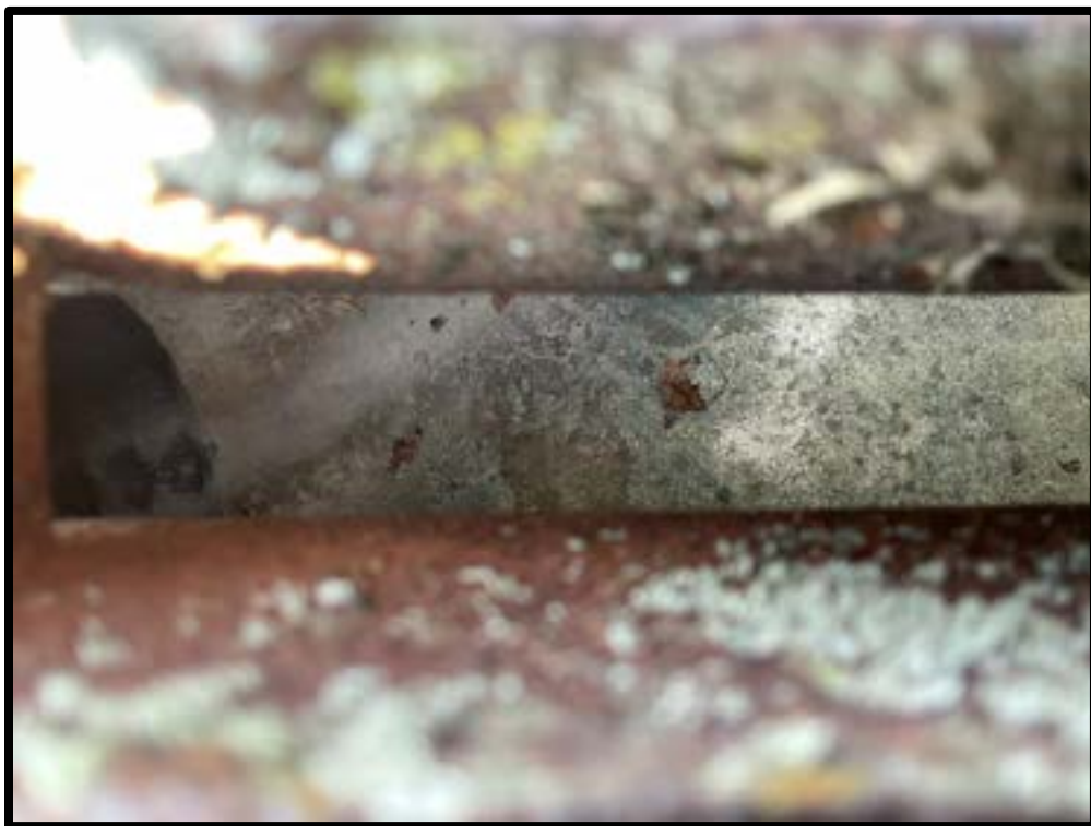
Photo # 1: Inlet grate seems to be in good condition
