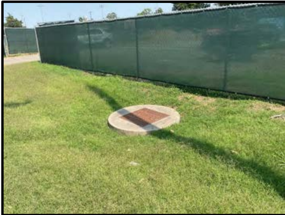
Photo #1: Grate inlet
