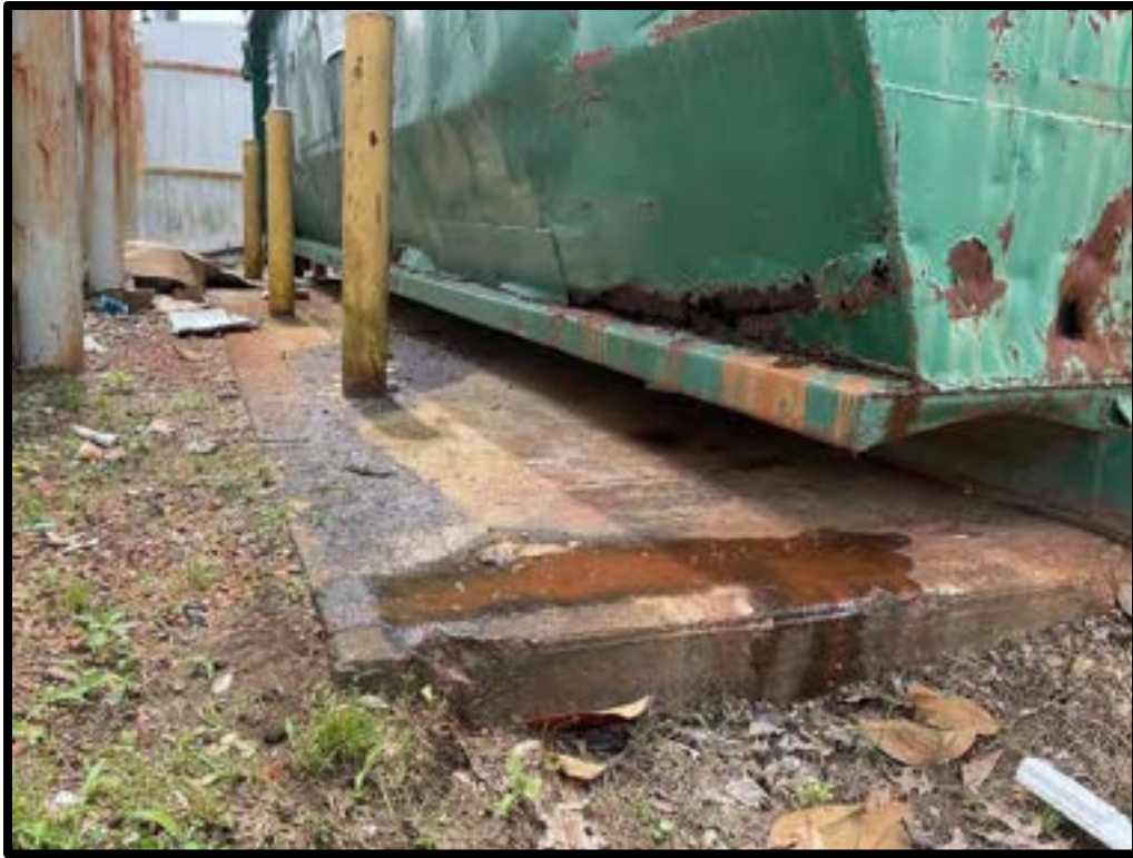
Photo #8: Active discharge from dumpster
