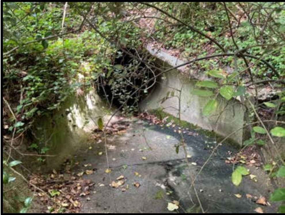
Photo #1: 24" Concrete pipe
