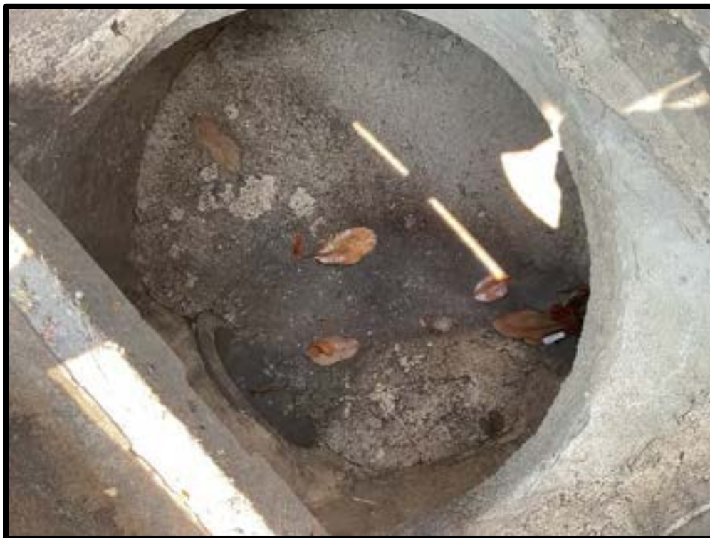
Photo #2: Minor sediment accumulation present
