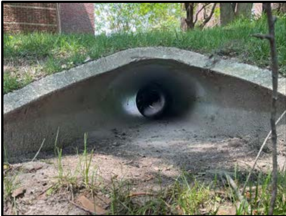
Photo #6: Sediment and vegetation accumulation present in northern inlet pipe
