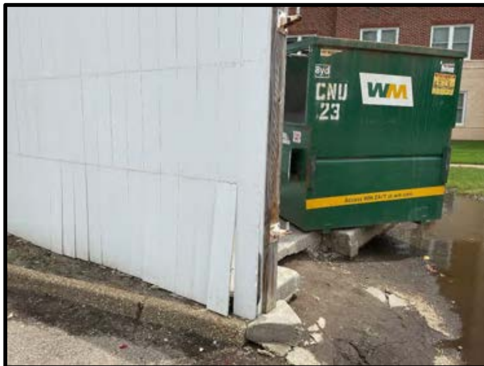
Photo #3: Damaged secondary containment and concrete pad
