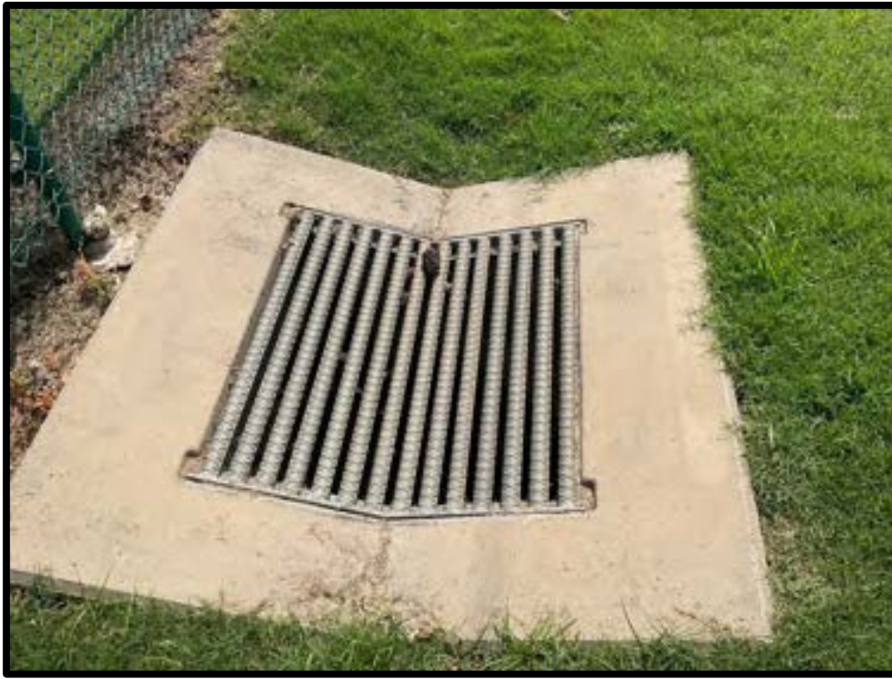
Photo #1: Grate channel and grate inlet
