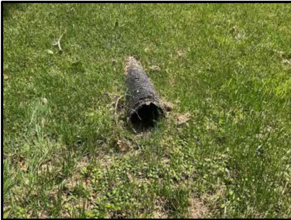
Photo #5: Sediment and vegetation accumulation present in southeastern roof drain
