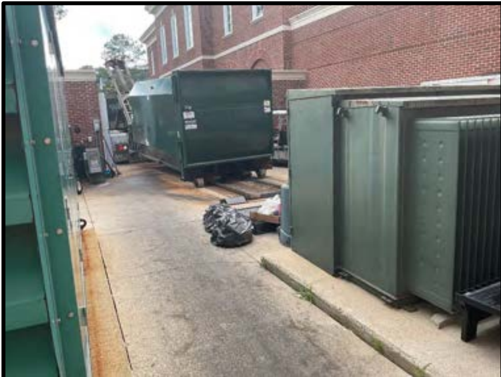
Photo #8: Trash compactor replacement during inspection
