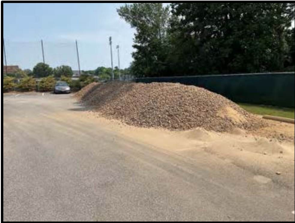
Photo #1: Uncovered stockpiles
