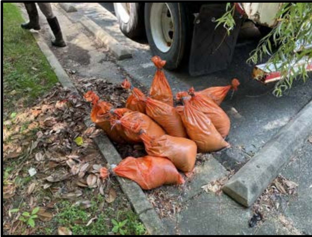
Photo #6: Sandbags storage present near BMP
