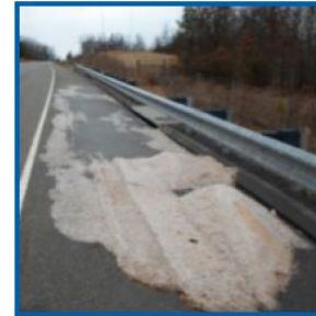
Mismanaged / Excess Road Salt
